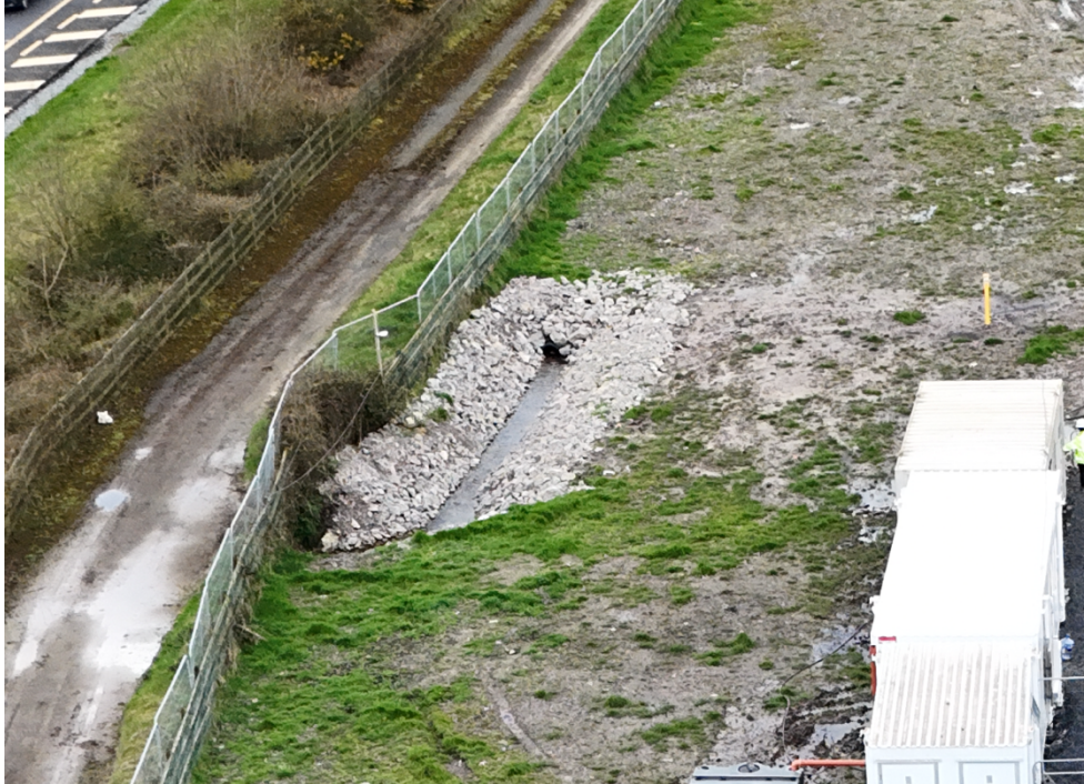
Plate 1 – Rip-rap section on Site Drain_01
